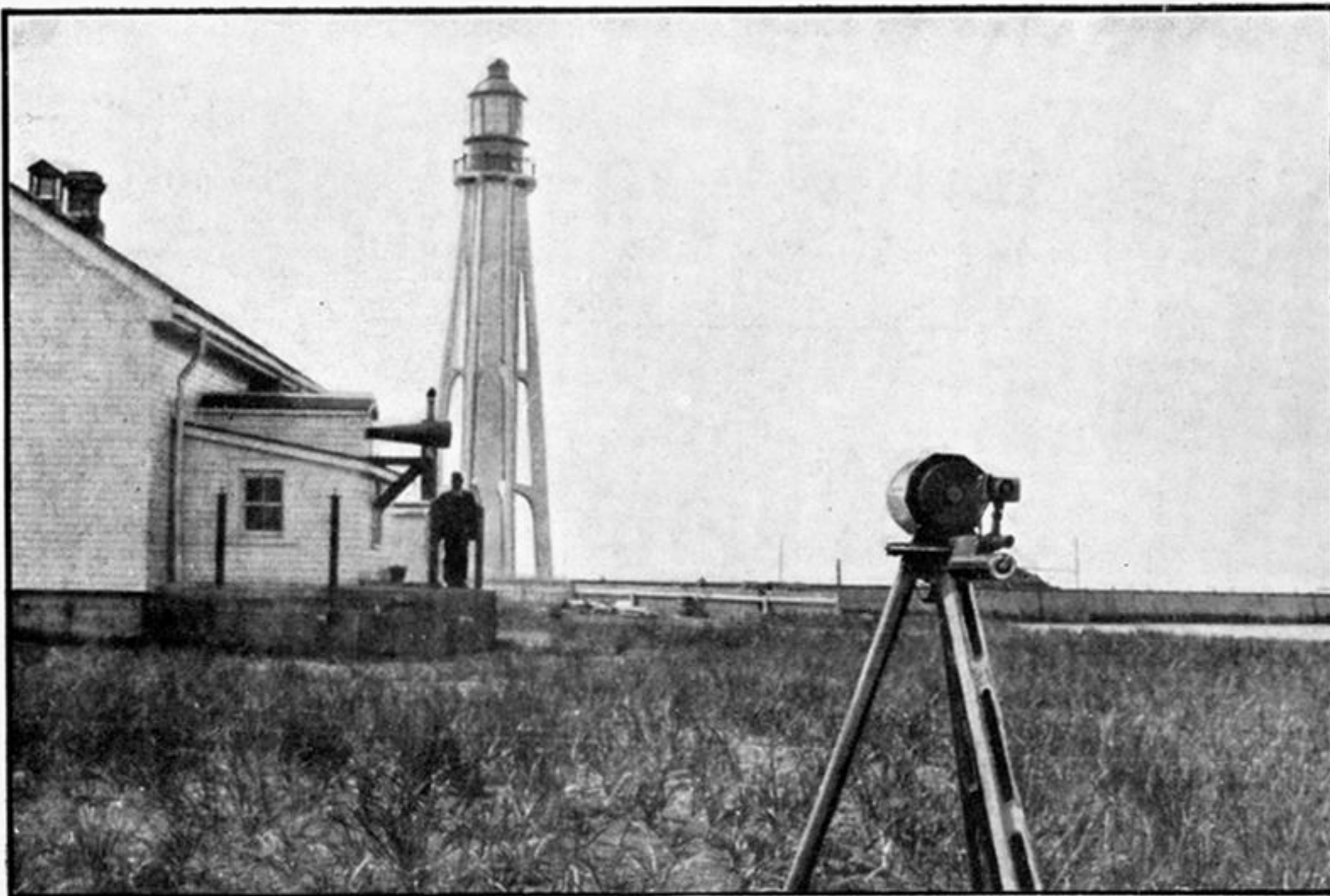
(i.) Webster phonometer mounted on a theodolite tripod. Building on the left is the fog-signal station, showing trumpet of diaphone. Father Point lighthouse in the background. The results obtained are shown graphically in Chart 1.
